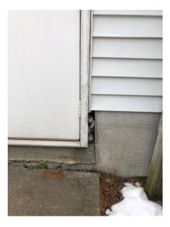
**46:** The foundation and footings are unreinforced brick and mortar. This system is not designed to withstand seismic forces. The existing installation has performed adequately to date, but consideration should be given to eventual replacement.
