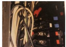
**9:** Multiple wires are installed on individual terminals. This 'double lugging' is not permitted because positive connection for all wires is not assured. We recommend reconfiguration of the circuitry so that each wire connects to only one terminal.
