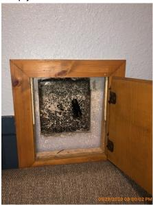
**30:** The fireplace does not have a damper. The glass doors across the fireplace may be used in lieu of a damper to minimize interior heat loss when the fireplace in not in use.
